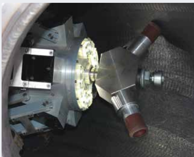
Sandblasting using JettyRobot
