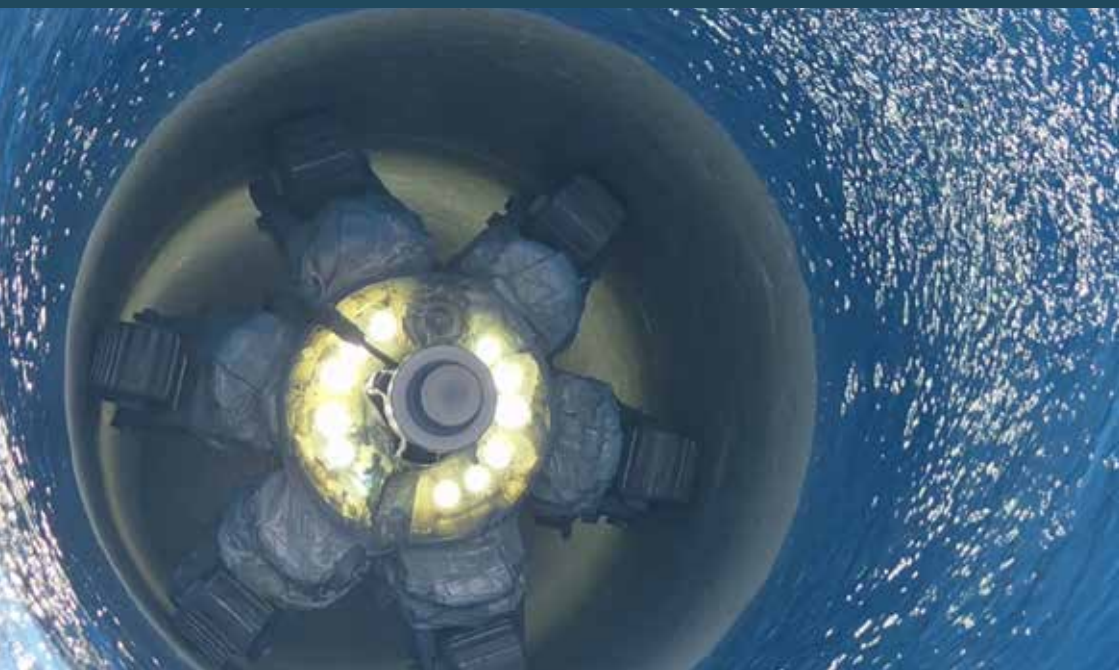
Internal coating of pipe using JettyRobot
