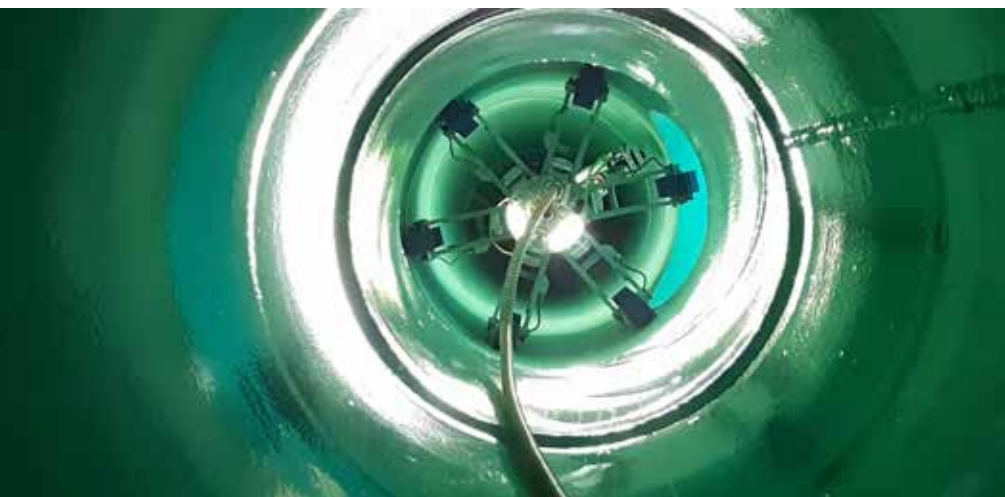
Internal coating using JettyRobot
